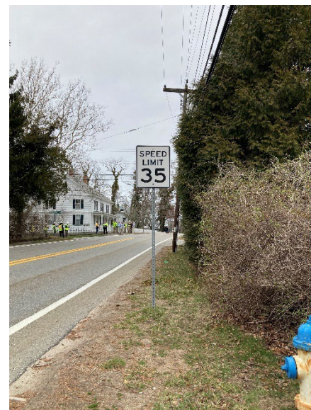
Image 7: Speed Limit Sign on Route 28A at Chapoquoit Road, Facing North. Vegetation Obstructs This Sign in Warmer Months
