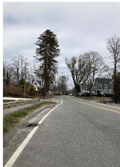
Image 13: Storm Drains on Route 28A As It Widens North of Old Dock Road
